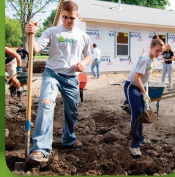
Students building a Habitat for Humanity house
