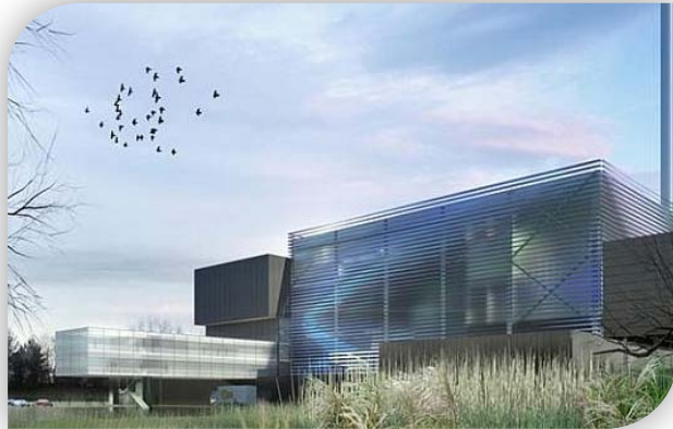
Powering 30,000 Homes Suffolk County, UK Sita UK Waste-to-Power Plant
